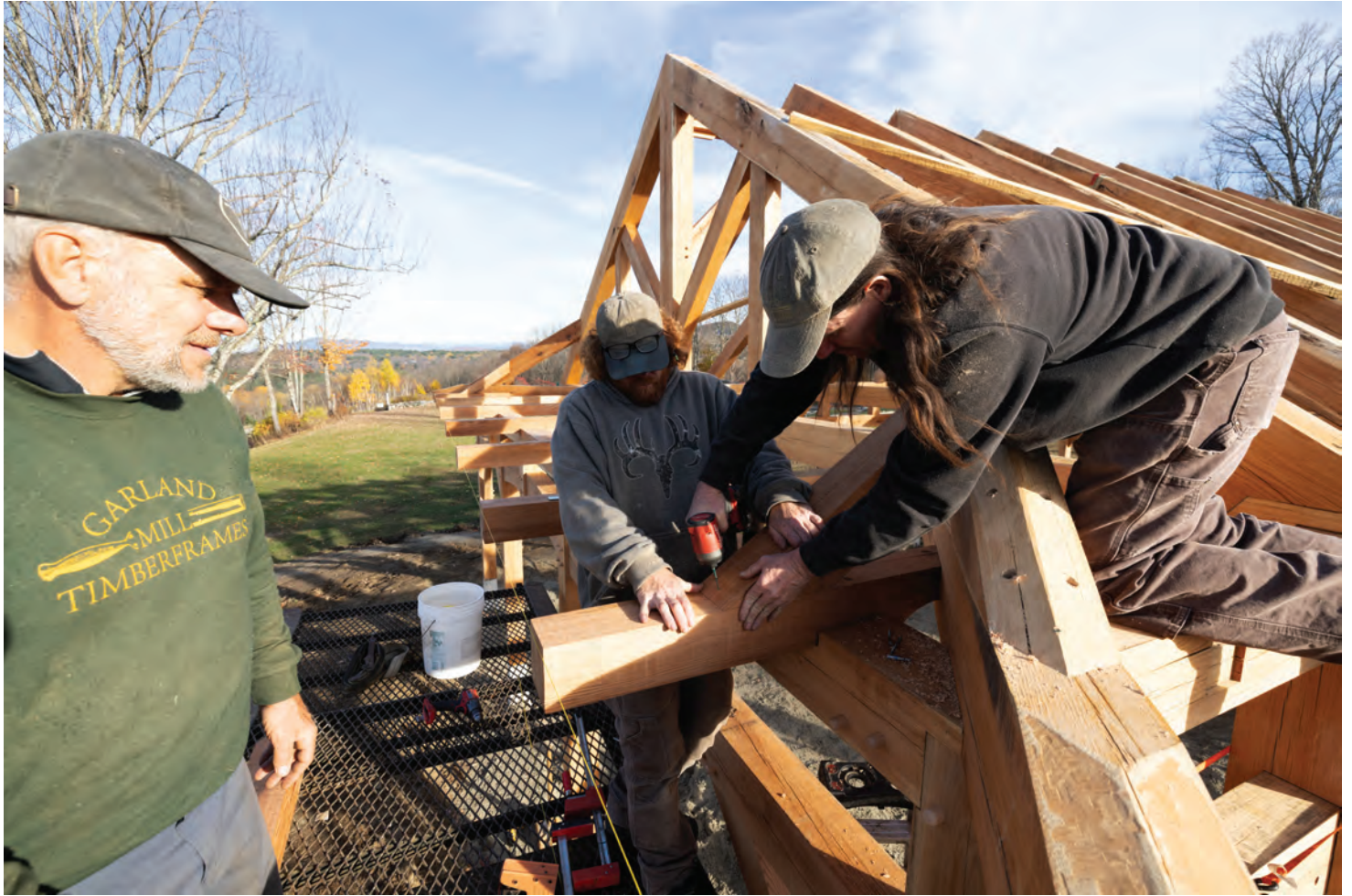
From left, Dana Southworth looks on as brothers Luke and Seth Colby install the gable-end structural rafter assemblies. These are attached to both sides of the diagonal corner “dragon beams,” and carry the curvilinear roof overhang that runs around the perimeter of the pavilion.
