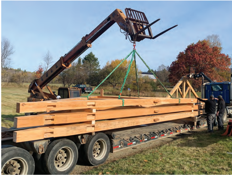
Carefully and methodically, crews load the 36-foot-wide king-post trusses onto a flatbed trailer for the journey from The Garland Mill in Lancaster to The Rocks in Bethlehem.
